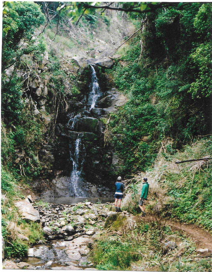
Max and Ash after restoring the track to Wairuru Falls.
